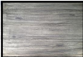
The natural aged “dock” allusion that extends out over the water was created by first troweling on McKrete Concrete Overlay (*patented acrylic and epoxy cementitious system*), adding a custom wood graining effect. Various colors of Chromastain (*environmentally-friendly/water-based/penetrating stain*) were then used to complete the unique decorative effect.
