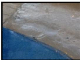
As for the “beach,” it also was troweled using McKrete; then, sponge finished, with real shark teeth, shells, and beach sand being added to give the look of a “real beach.” The floor was sealed with a protective coat of McKinnon Materials clear/UV resistant/100% solids Industrial Epoxy.
